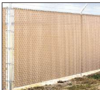
Look closely and you can see the round "noodles" which lock the slats in place at top and bottom.
