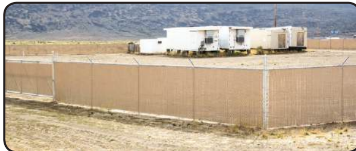
The above photo shows the recently completed equipment yard with the new PrivacyLink perimeter fence that provides privacy and security.
